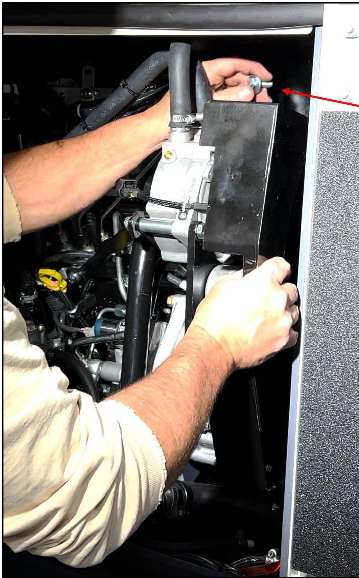
Install the LHG belt guard assembly (140-0146-A0 for 45kW, 140-0147-A0 for 25kW).
